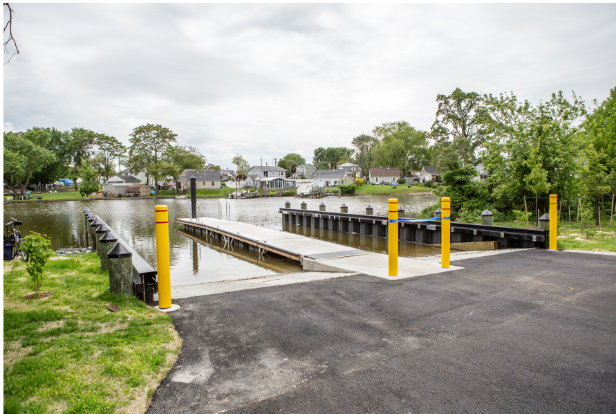
New 2-lane boat ramp at Merritt Point Park
